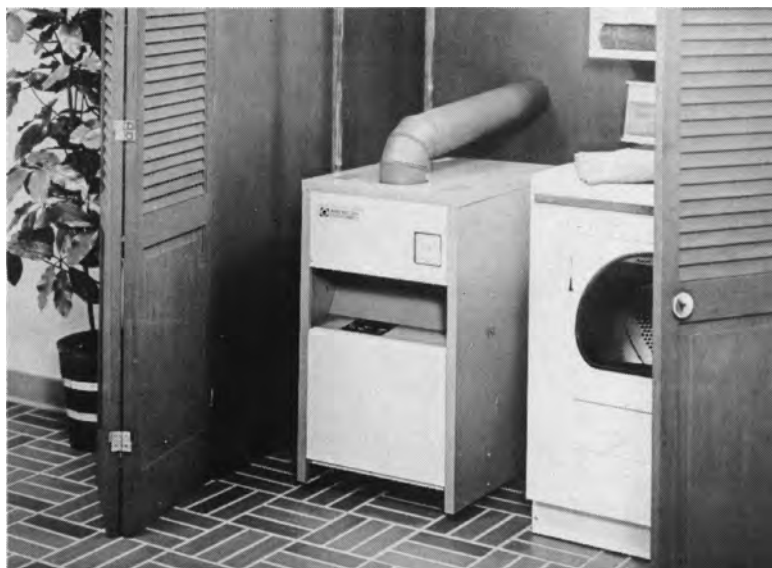
Figure 9-1 Electric-fired boiler. (Courtesy National Better Heating-Cooling Council)
