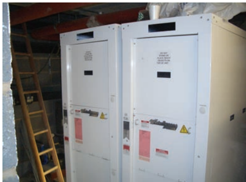
Figure 11. Central plant using water source heat pumps
