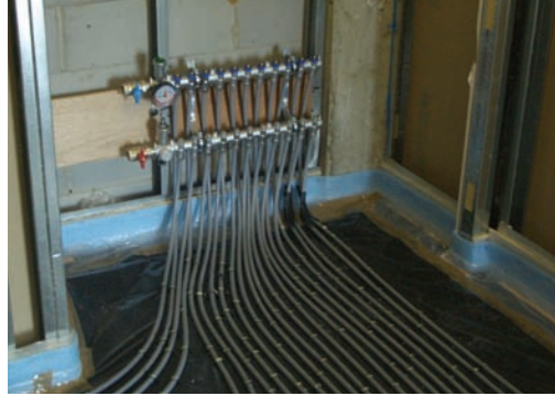
Figure 8. Manifold for radiant heating and cooling
