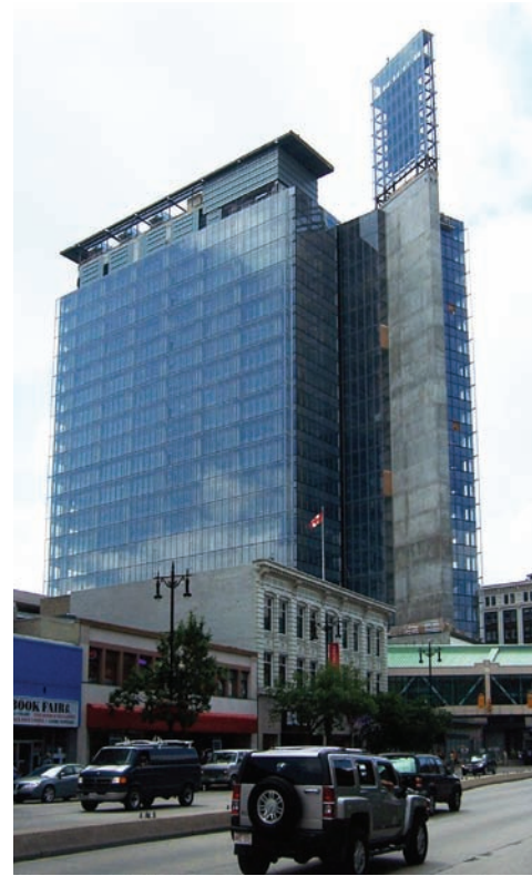
Figure 3. Thermal Chimney design at Manitoba Hydro
