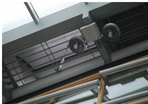
Figure 23. Mechanical roof vents in garden / atrium area
