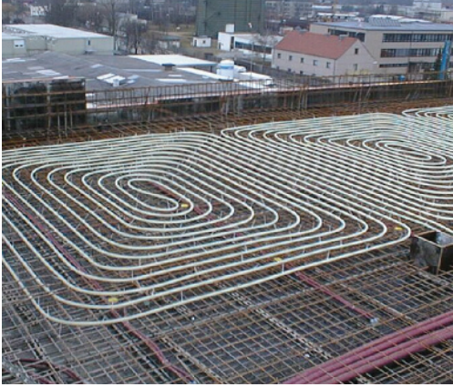
Figure 2. Thermo-active slab
