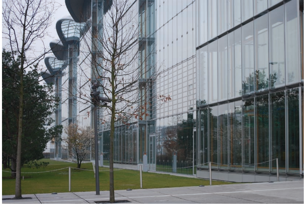
Figure 20. Lufthansa Aviation Center employs single and double- façades with mechanisms for natural ventilation and shading
