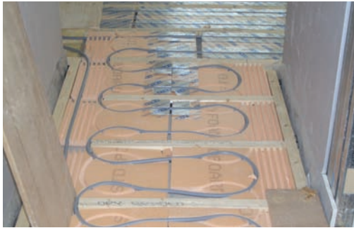
Figure 9. Tubing mounted in raised floor for use under carpet or hardwood
