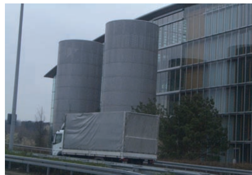
Figure 24. Outdoor air inlets – used for pre-conditioning of makeup air
