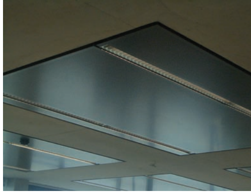
Figure 15. Convertible ceiling panels reserved for additional cooling/heating capacity
