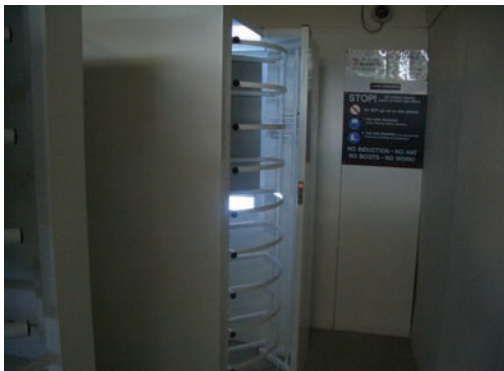
Figure 12. Construction site entrance – turnstile with facial recognition to verify identity and safety gear prior to entry to site
