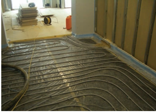
Figure 7. In-floor tubing for radiant heating and cooling
