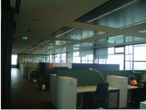
Figure 14. Office space with thermo-active ceiling slab and ceiling panels reserved for additional capacity
