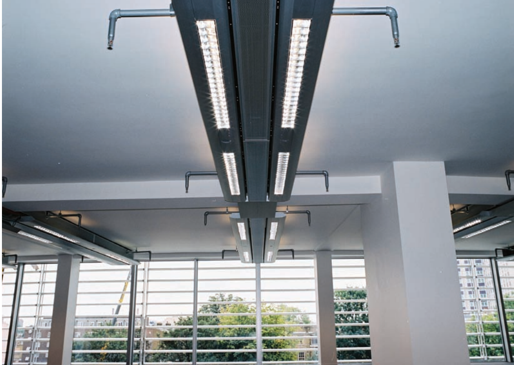
Figure 6. Active Chilled Beam
