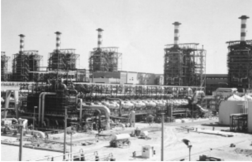
FIGURE 4.1.2 One of the six units of the 346,000 m 3 /day MSF desalination plant Al Taweelah B in Abu Dhabi, United Arab Emirates. (Courtesy of Italmimpianti S. p. A.) It is a dual-purpose plant, composed of six identical power and desalination units. Five of the six boilers are seen in the background. The desalination units were in 1996 the largest in the world. They have 17 recovery and 3 reject stages and a performance ratio (PR) of 8.1. The plant also produces 732 MWe of power.
